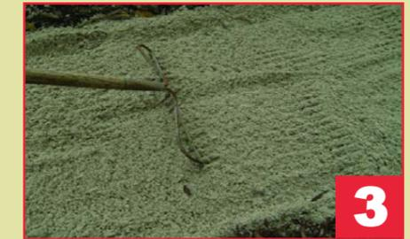
Add about two inches of sand and smooth it out to make a stable but pliable base for the stone. Without sand, the pathway would be less stable and the stones would be prone to cracking.
