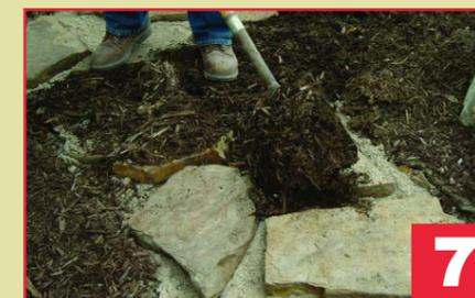
Fill the area in between the stones with mulch, gravel or sand. Sweep the filler material into all of the gaps. Thoroughly water the pathway to wash the stones and help them and the material settle.
