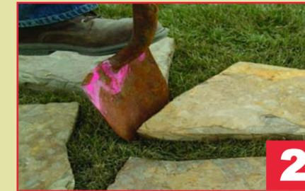
Once the flagstones are in their permanent spots, cut into the sod and around them with a sharp shovel to mark the shape. Remove two inches of soil plus the depth of the stone to make room for the base material and the stone.
