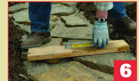
Lay a 2x4 board across the surface of the flagstone and tap the board with a rubber mallet to seat the flagstone firmly in place. Double check the level of the stones.
