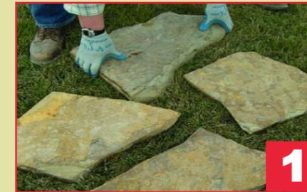
Place the stones where you think they will work best. Arrange them so the spaces between them provide a comfortable stepping distance. Adjust the stones to create gradual curves if desired. Walk the path in both directions a couple of times and make any final adjustments.
