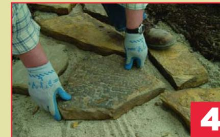
Place the flagstone into the layer of sand or other base material and gradually twist the stone into place. Stones should not rock or teeter.
