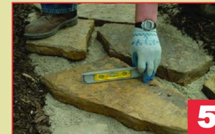
Check to make sure the stones are level to the ground. If they aren't, adjust the sand and stone accordingly.
